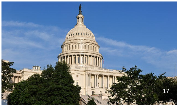
Figure 19. Capital Dome, Washington DC 28 .
